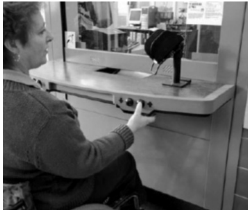
Photo 9. Ticket box office example that can be lowered (DFT, TScot, 2008)
