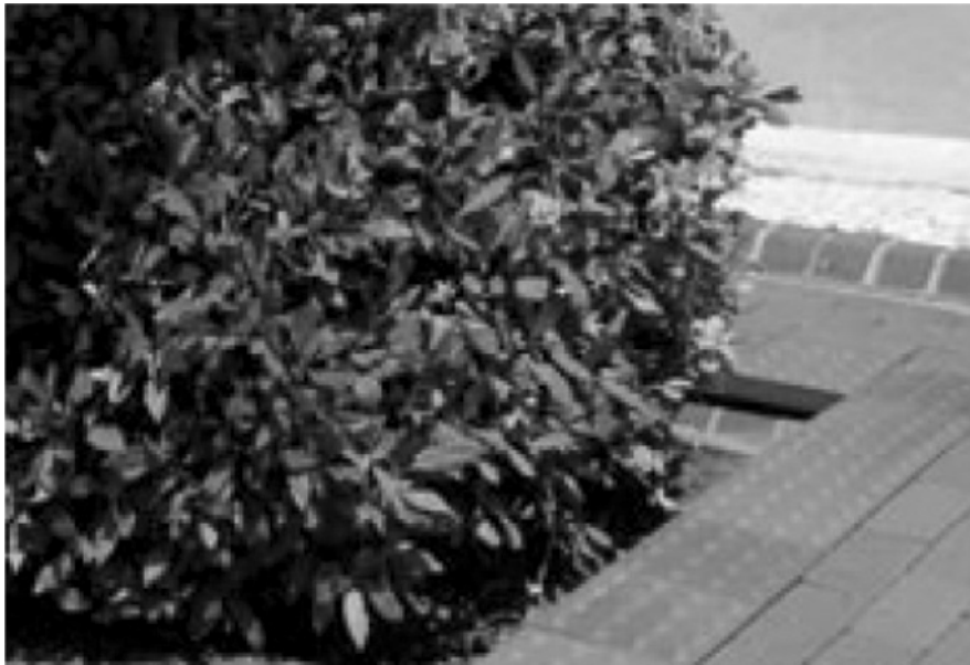
Photo 17. Warning with walkway flooring against objects
